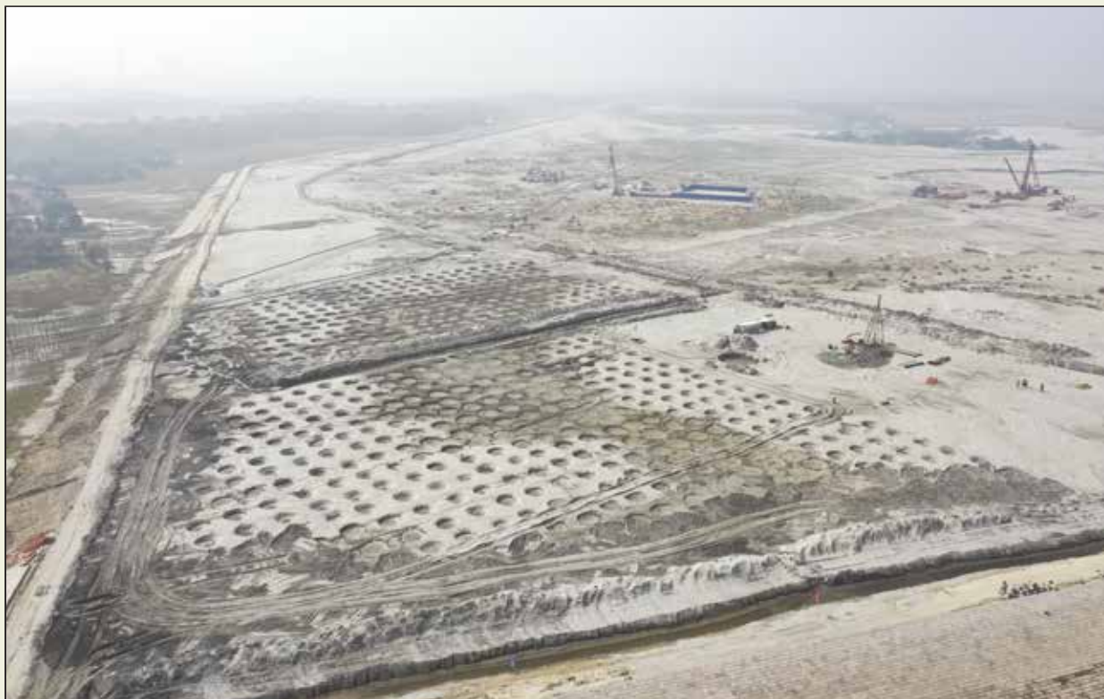
Dynamic Compaction Work at Temporary Office and Living Area
