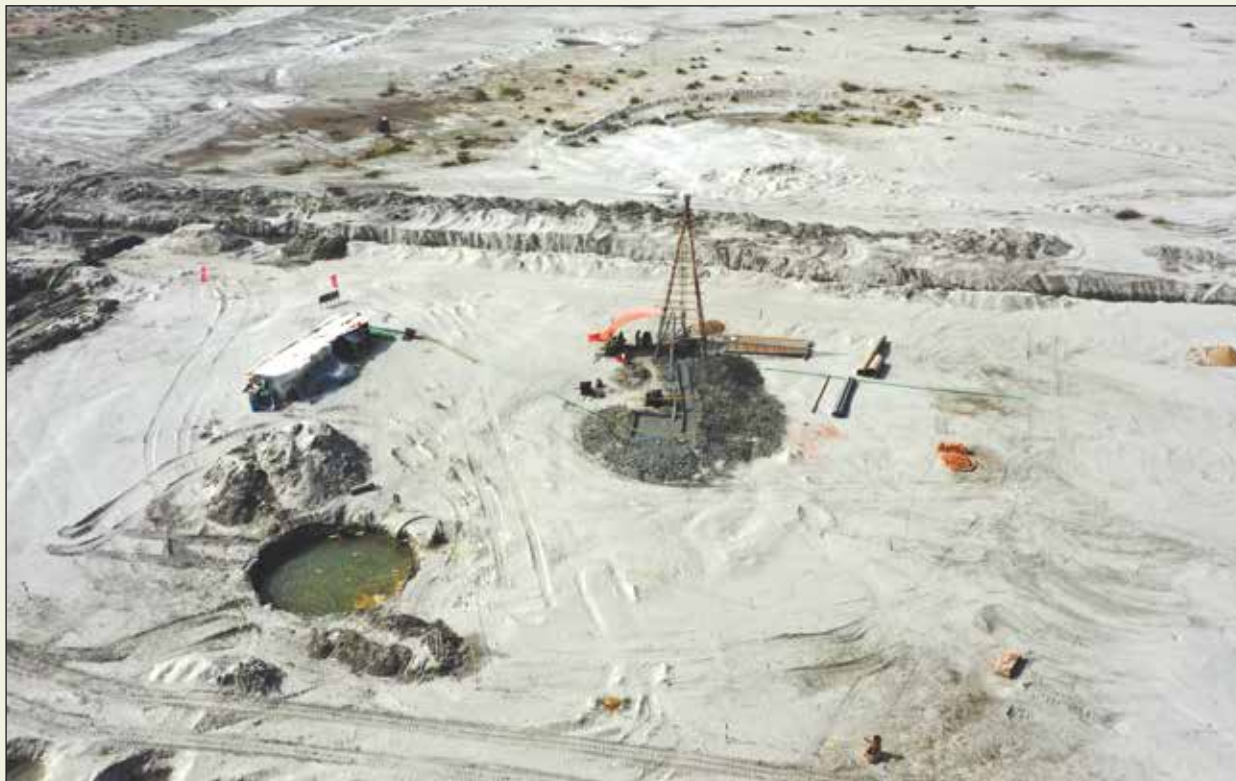
Deep Tube Well Construction at Project Site
