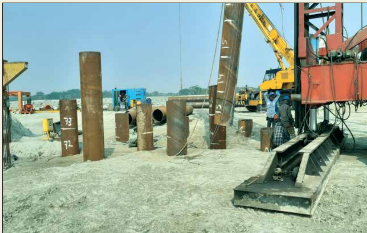
Steel Pipe Pilling Test Activities at Main Power Block Area
