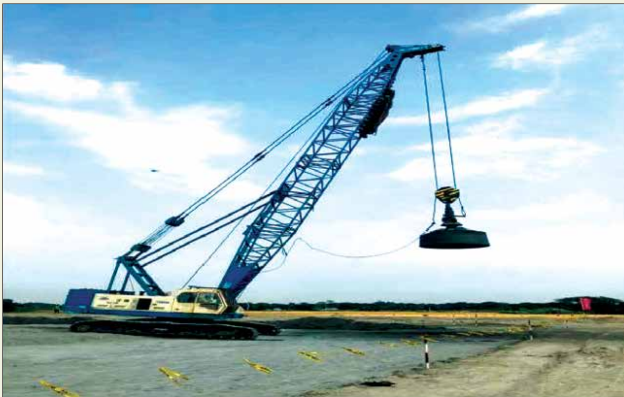
Dynamic Compaction Work at Batching Plant Area
