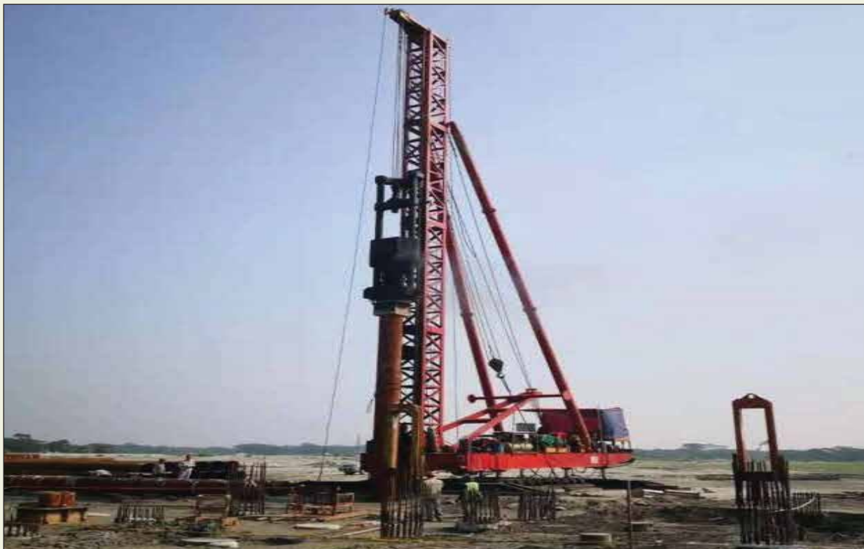
Steel Pipe Piling Test at Main Power Block Area of Project Site
