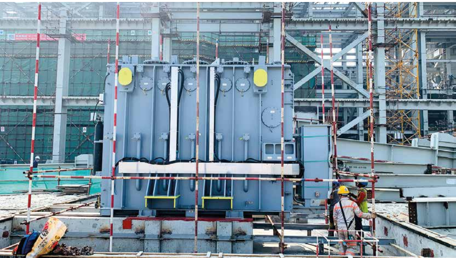
Unit Axiliary Transformer Installed at Power Plant Site
