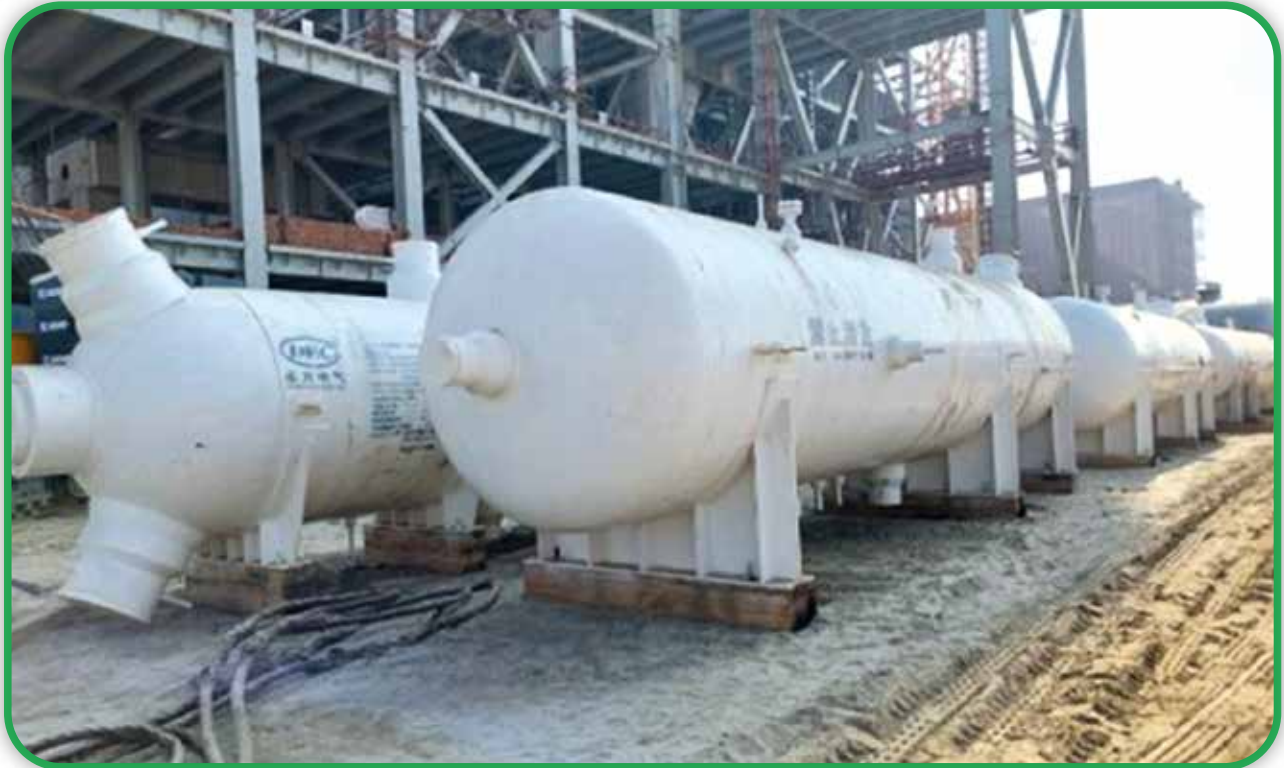
Steam Turbine - HP Heater and LP Heater installation works at Power Plant Site
