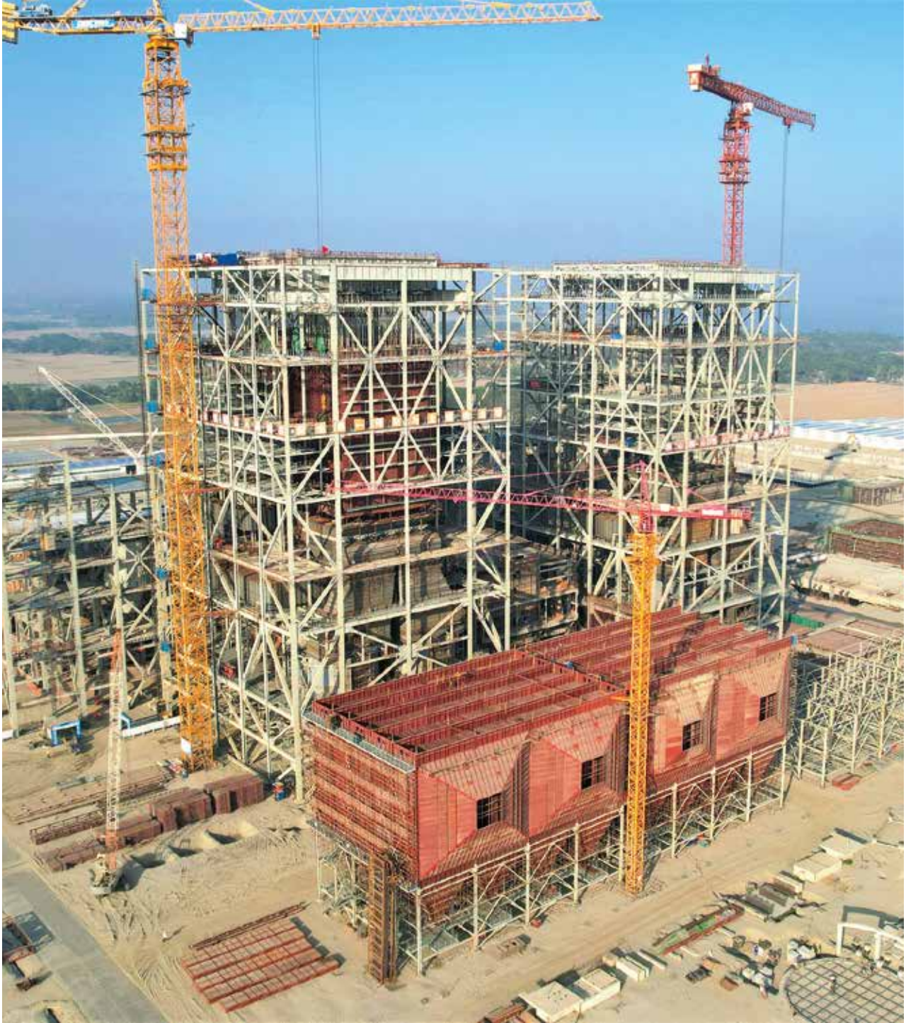
Boiler Super Structure
