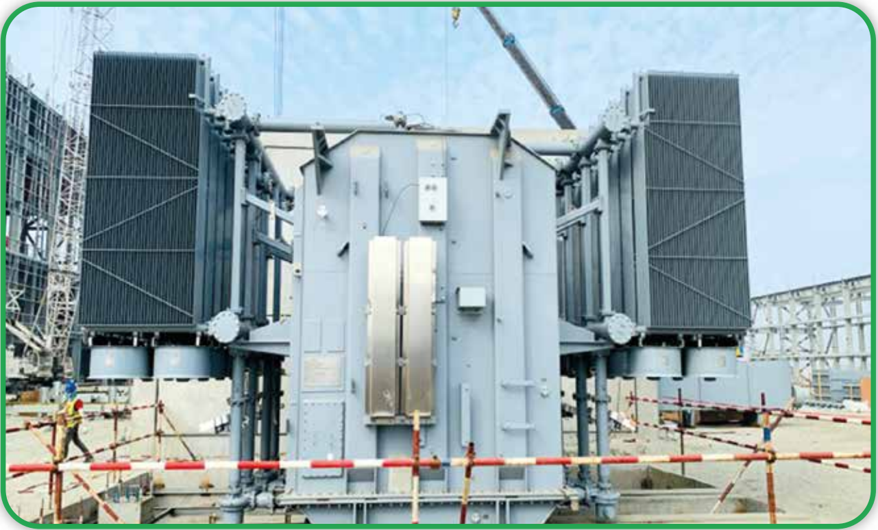
270 MVA Main Transformer Installed at Power Plant Site
