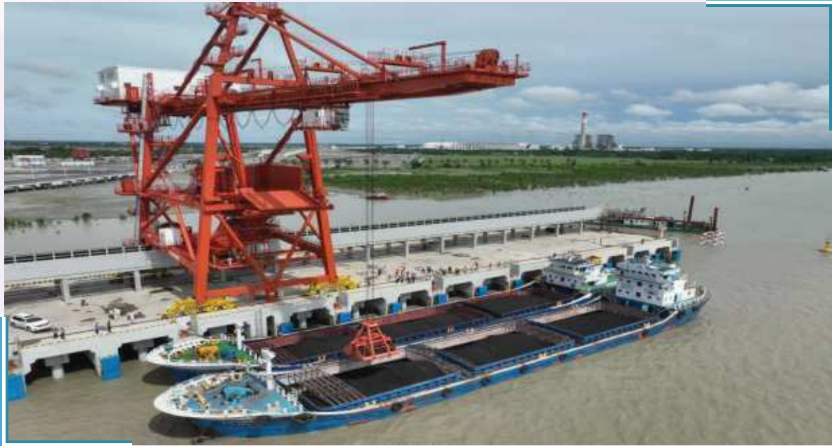
Coal Unloading at Jetty Area
