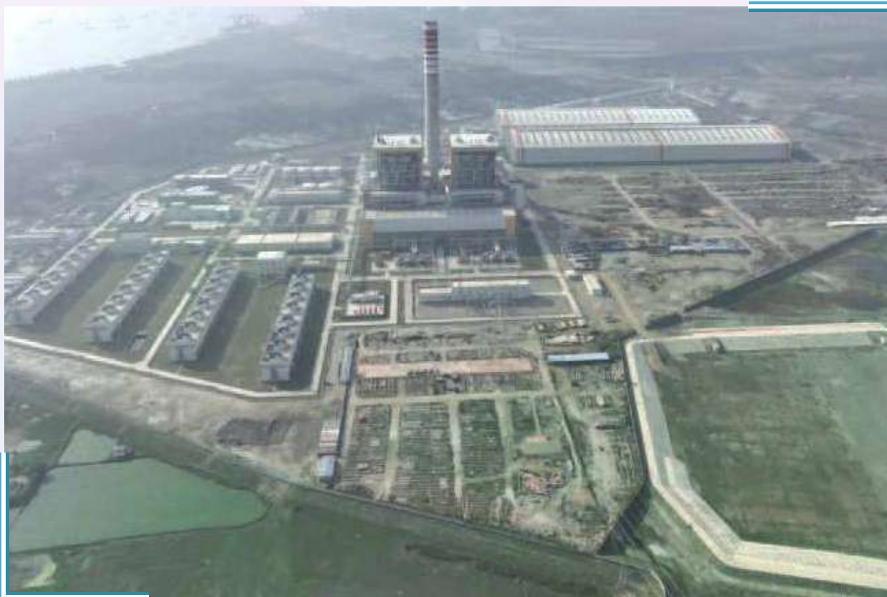
Bird's Eye View of the Project
