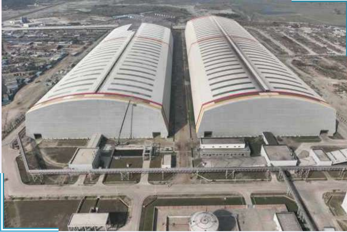
Coal Storage Shed
