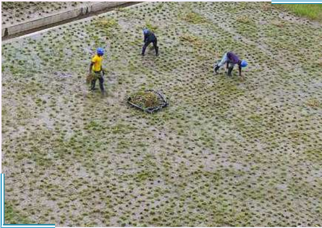
Landscaping Work at Project Site
