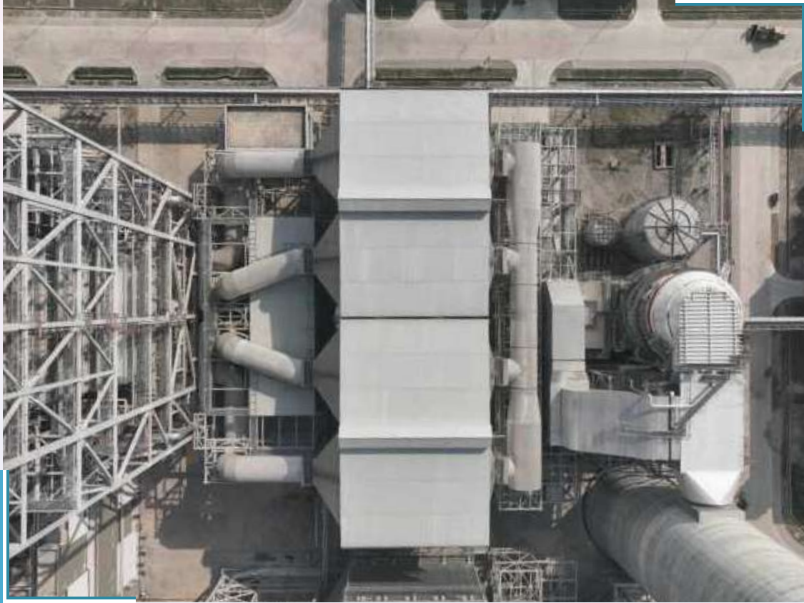
Electrostatic Precipitator of Boiler
